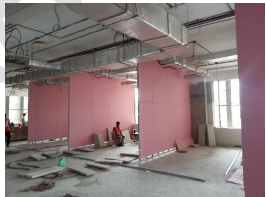
Figure 5.10 Insulated ducts
