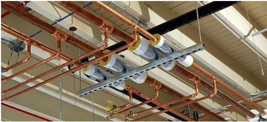
Figure 5.8 Chilled water pipe insulation installation
